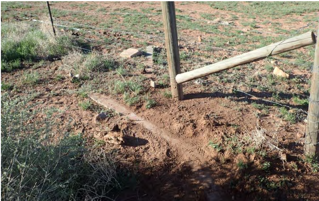
Figure 5-7. Previously unrecorded concrete features associated with the historic irrigation ditch (42GR3625).
