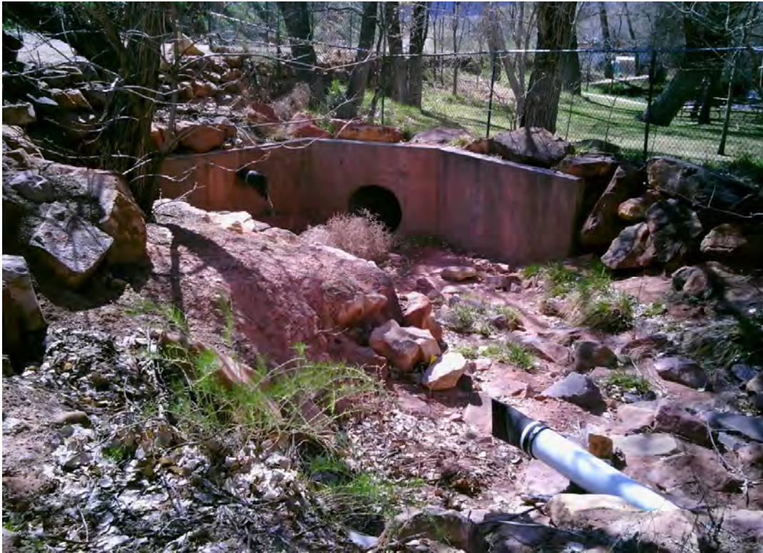
Figure 7 – Channel Mapped as Dry Wash Below Detention Basin
