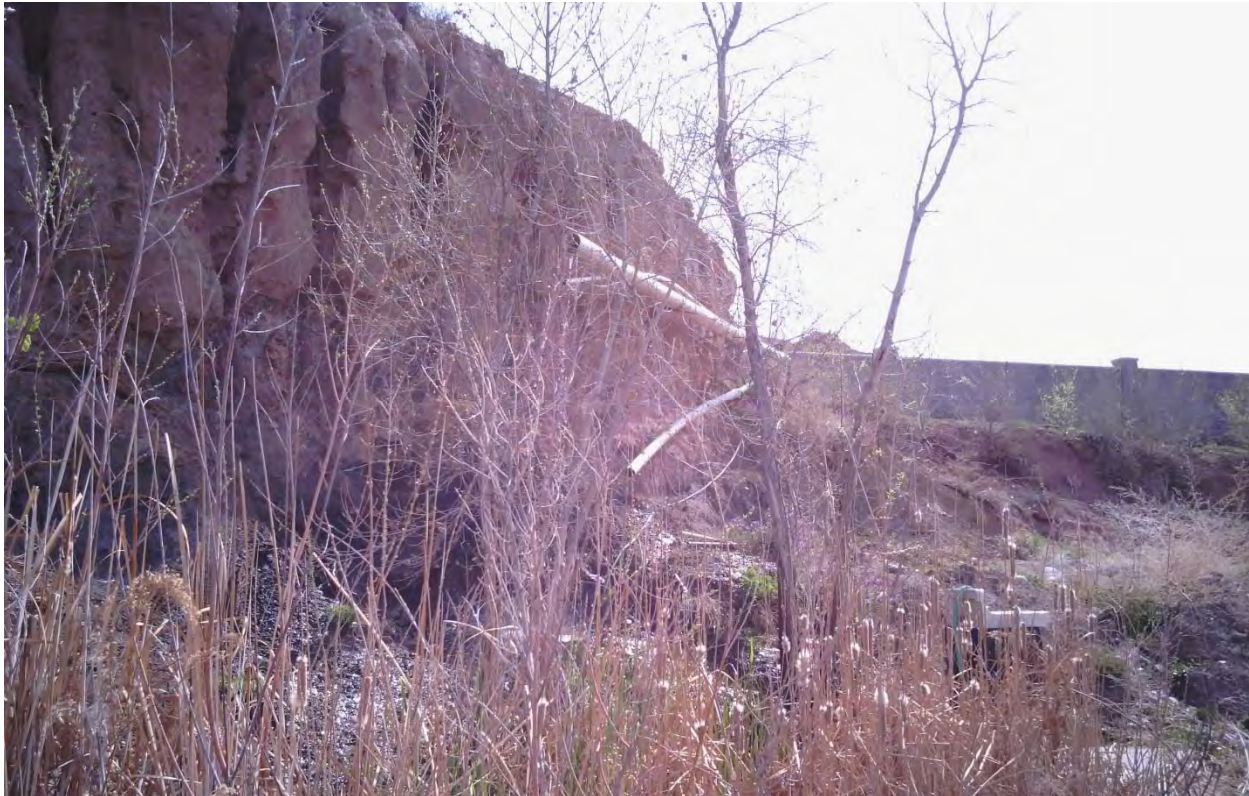
Figure 12 – Discharge Pipe from Ornamental Pond
