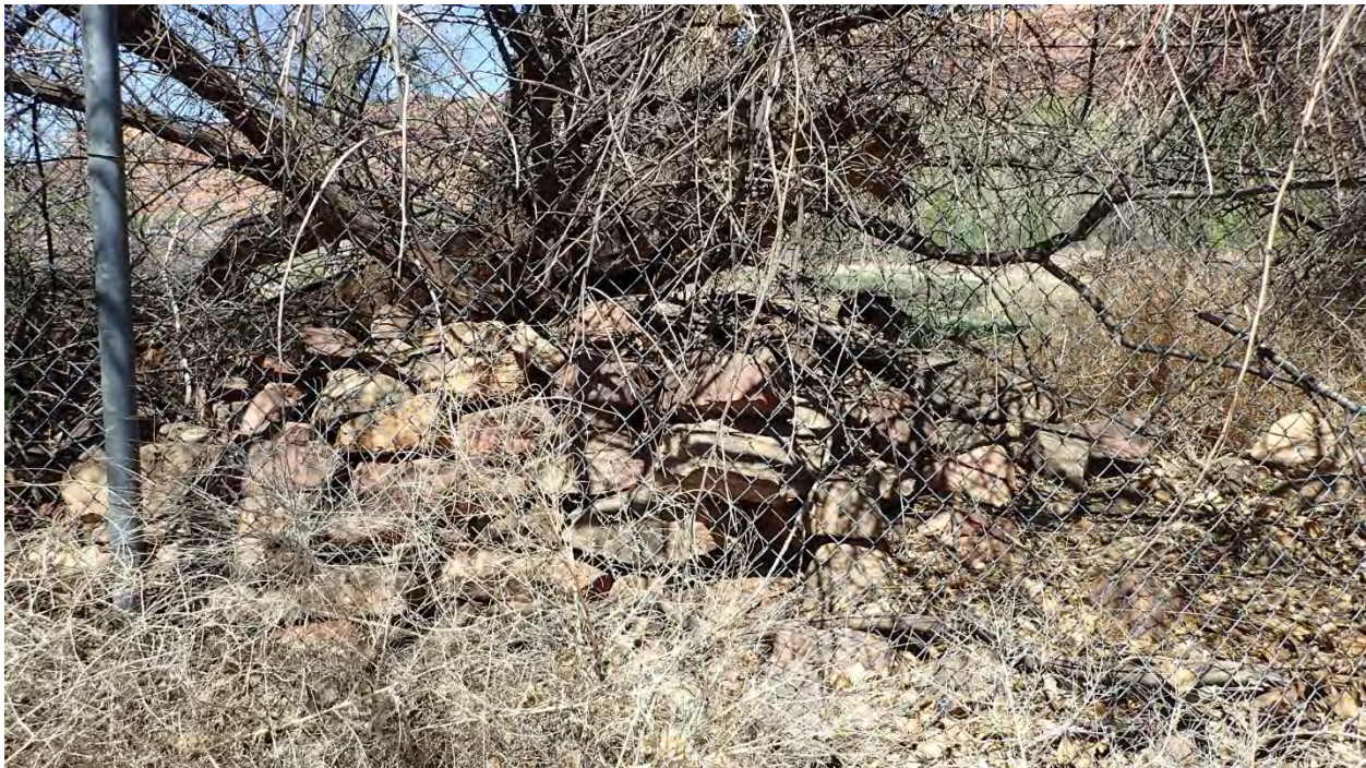
Figure 5-13. Overview of south wall of Elk Mountain Mission Fort Site (42GR5569).
