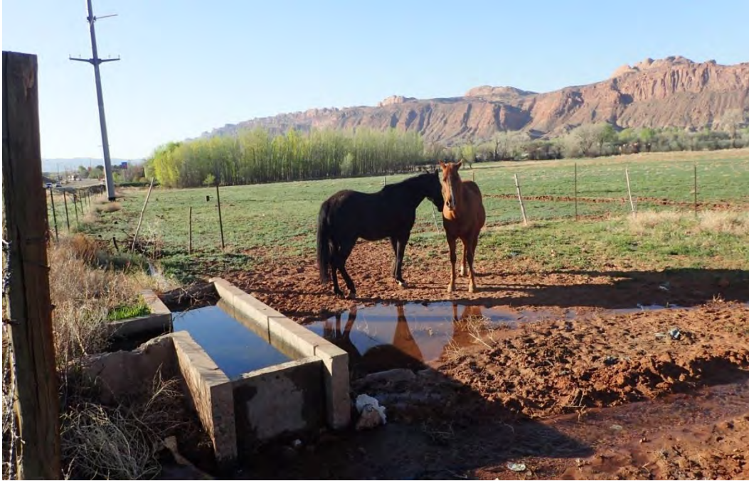
Figure 5-6. View of the headgate (Feature A) of the historic irrigation ditch (42GR3625), looking south. The ditch to the south (running just west of powerline) has been replaced by 10-inch PVC pipe. Note hand-dug feeder laterals in agricultural field west of the enclosure.
