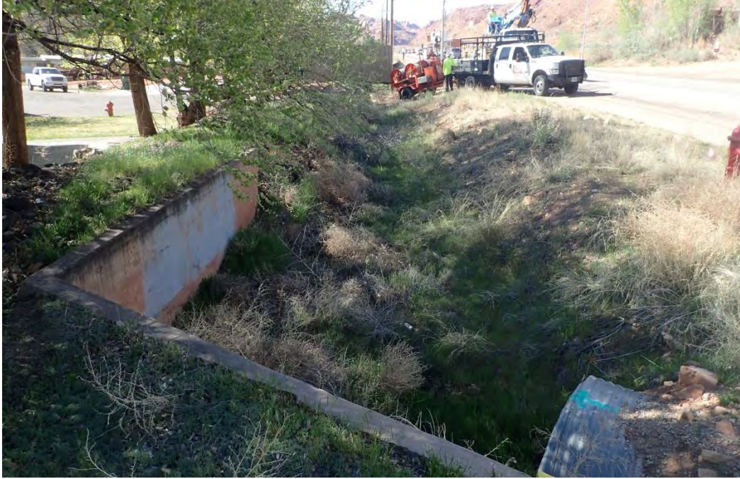
Figure 5-5. Feature B, concrete wall and culvert, for historic ditch (42GR3623).
