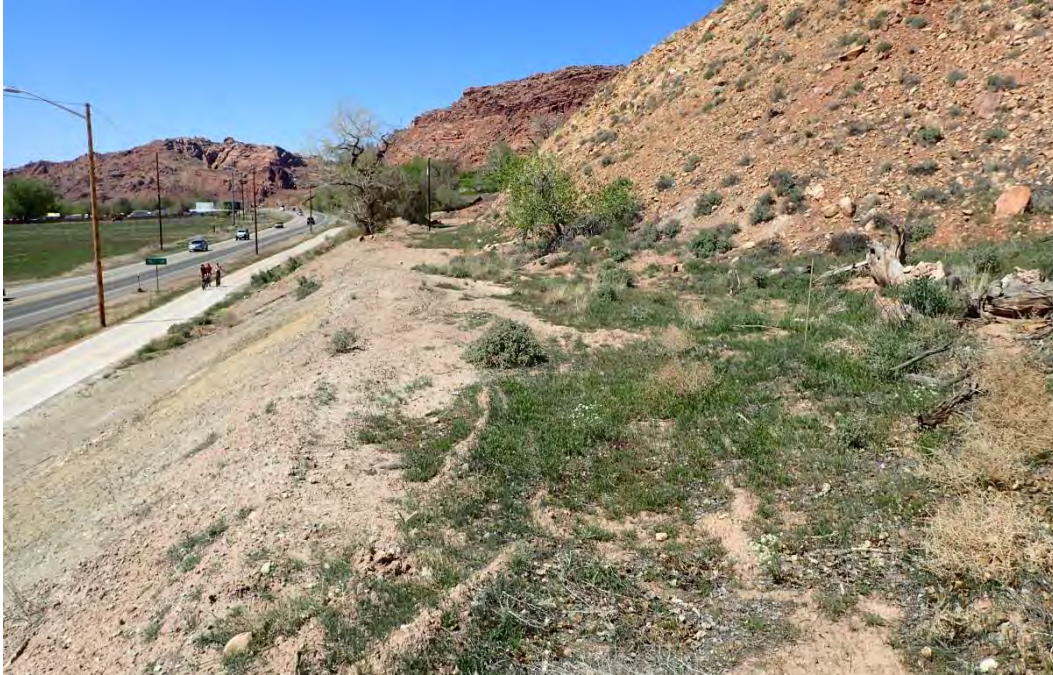
Figure 5-2. View of southern recorded segment of historic Moab-Thompson Wagon Road (42GR2813), looking north. Site destroyed by construction of bike path.
